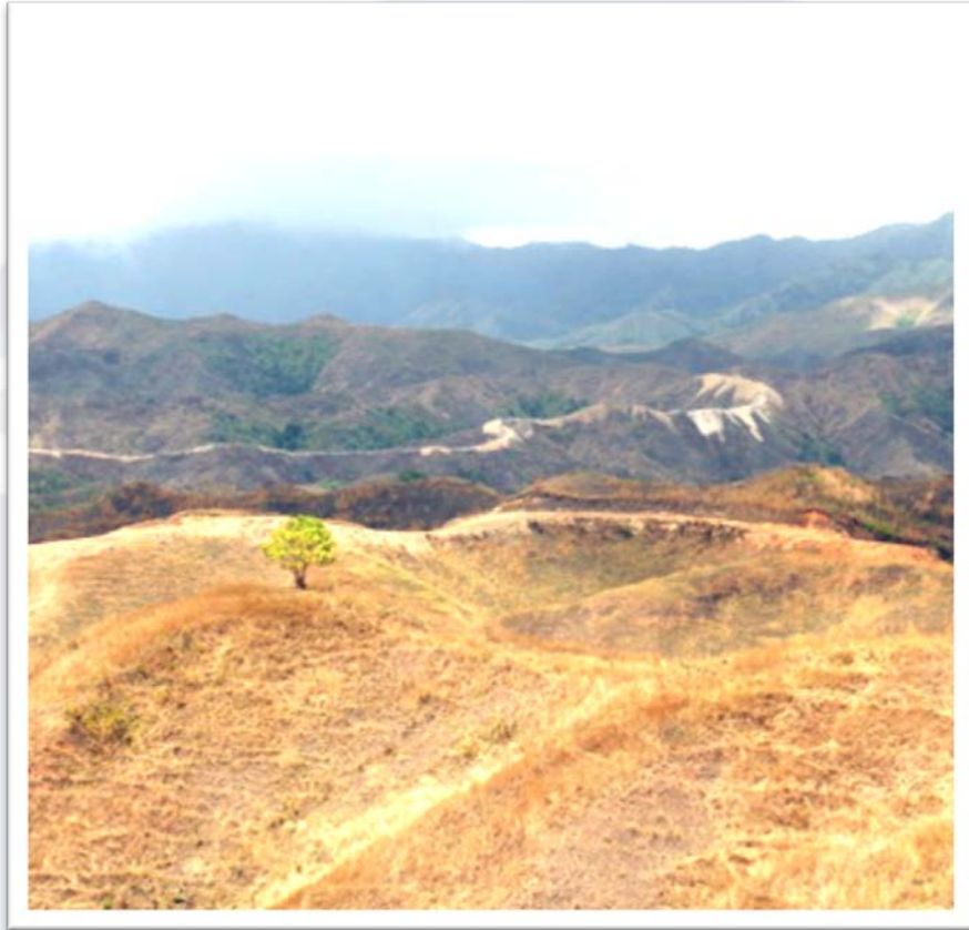
New 2.5 km access road to Nakoro drill site
